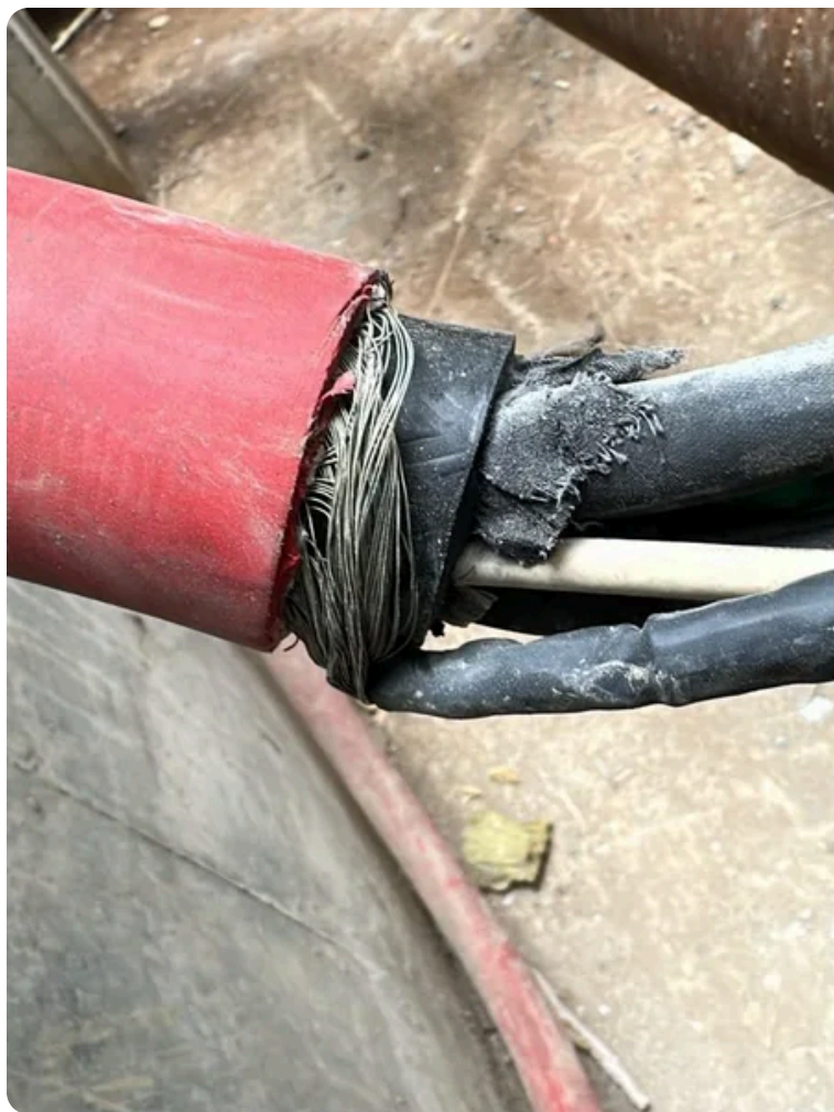
The cable being replaced: its stripped end (left) and its terminated cores (right). Photos: taken on site.
