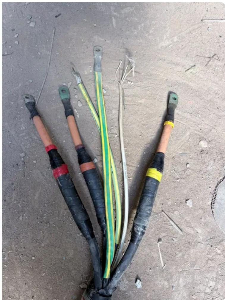
The cable being replaced: its stripped end (left) and its terminated cores (right). Photos: taken on site.
